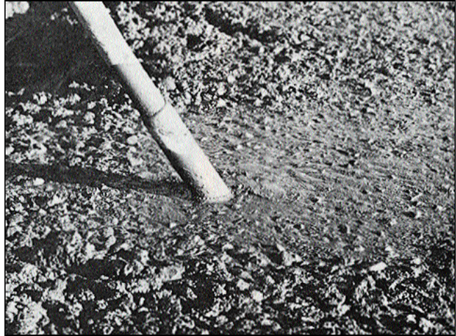
Figure 1. Internal vibrator liquefying low slump concrete.
