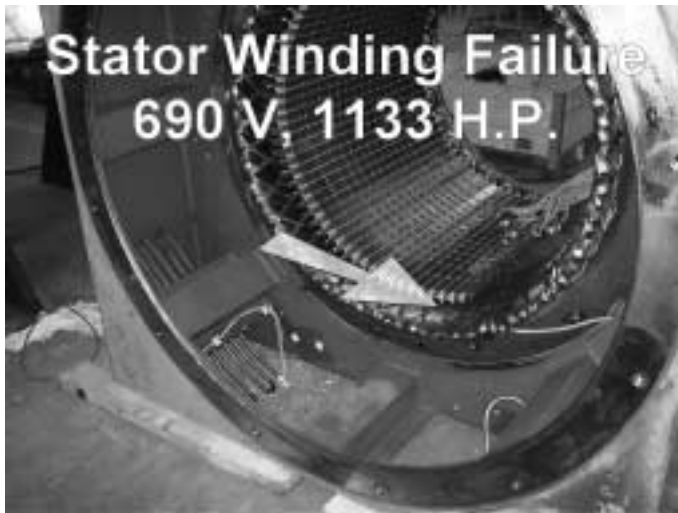
Figure 5: Picture of Motor 1 After Failure
