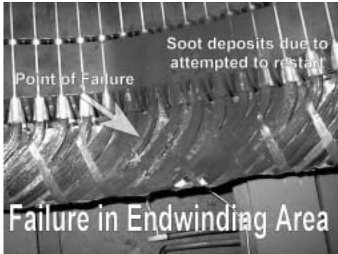
Figure 6: Close up of Motor 1 Failure
